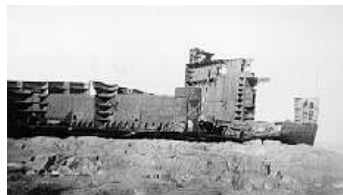
Figure 18 A considerable amount of salvage work has already been undertaken
