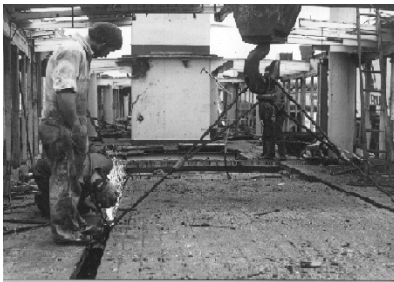
Figure 6 Workmen salvaging parts of the Bellubera before she was scuttled
