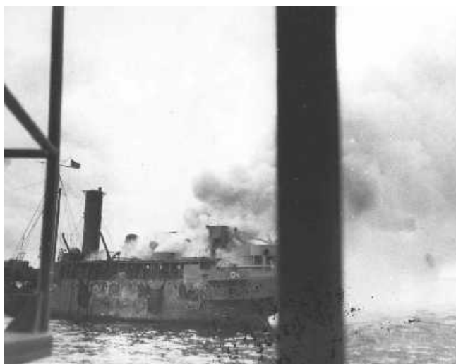
Figure 61 - The stern of the Kanawha shows the severe damage to engine room
