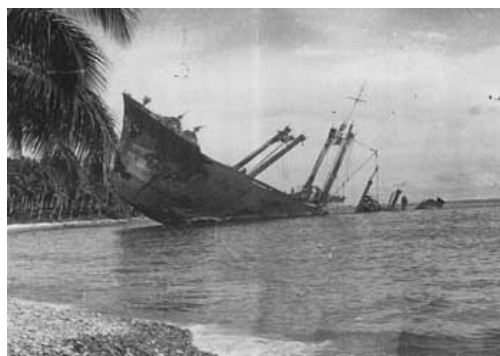
Figure 79 - Shot of the Kyusyu Maru from the opposite direction, taken 1944
